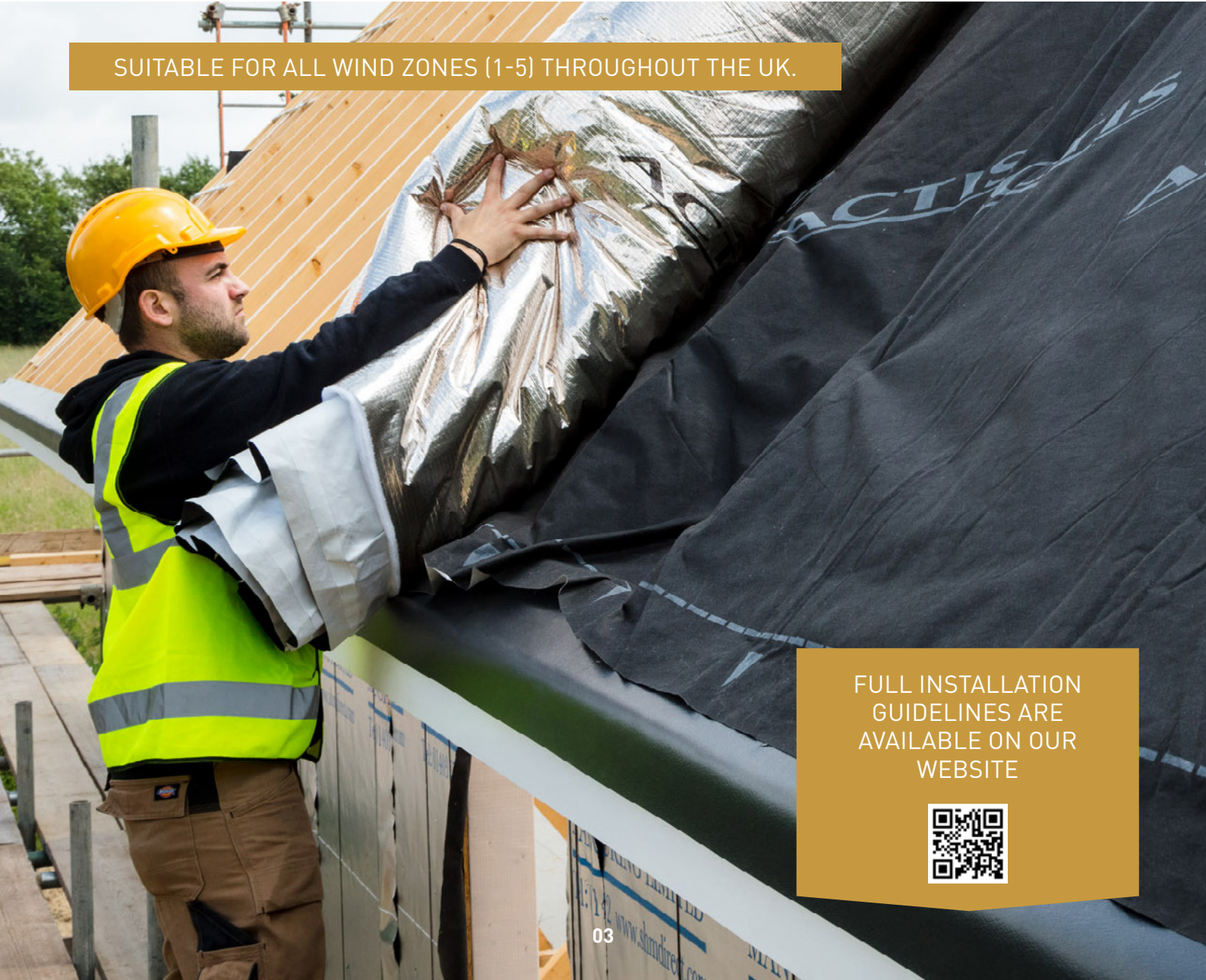
Boost'R Hybrid Roof as a substitute for Roof Underlay.
